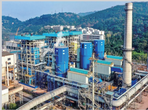
Chongqing Iron & Steel's Self-generating Energy Equipment
